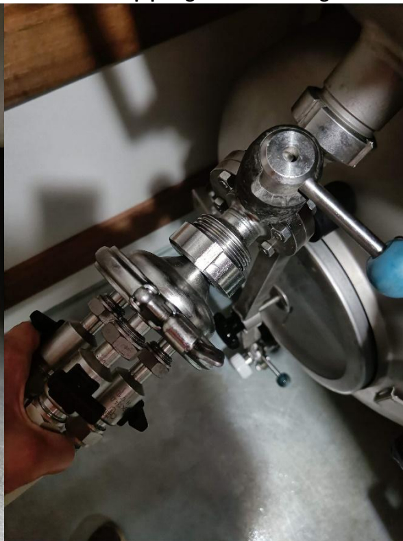
5. Attach the pipe again and hand tighten it
